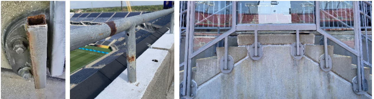
Existing Steel Conditions
